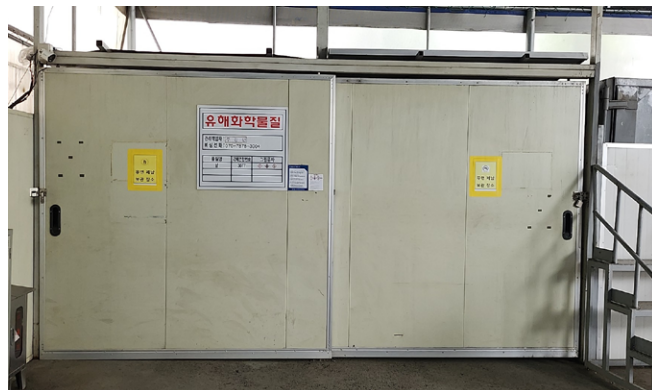
Waste treatment facility
