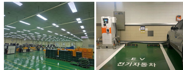
Installation of LED Lighting at Gyeongju Plant
